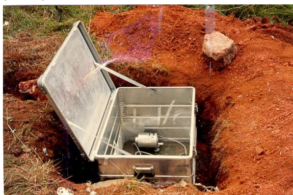
Photo 3. Seismometer installation at Dundu site.
